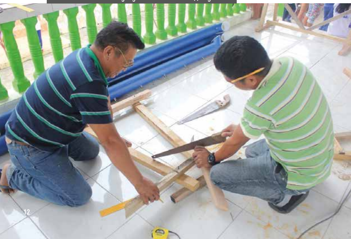
Members of PTA building legs for WASHaLOT 3.0 // Figure 10
