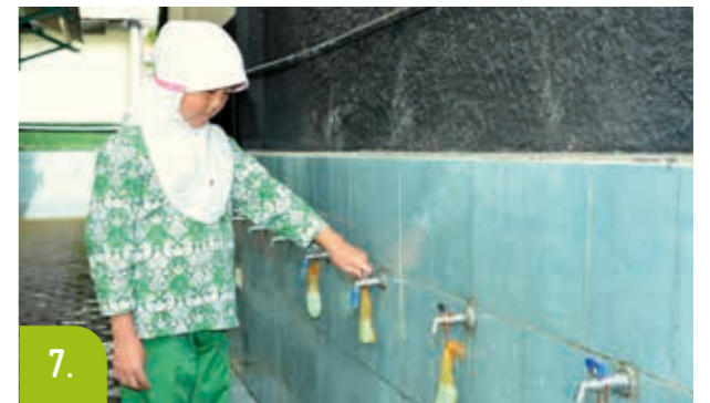
7. Fix dripping water pipes and faucets.
