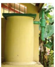
Attach the fabricated rain diverter to the existing PVC Drum reservoir. Align the position of the rain diverter when connecting it to the gutter down pipe and PVC drum inlet to maximize the flow of water into the reservoir.
