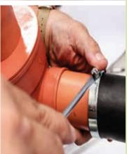
Install part # 6b with part # 7b to part # 4a. Tighten part # 7b.
